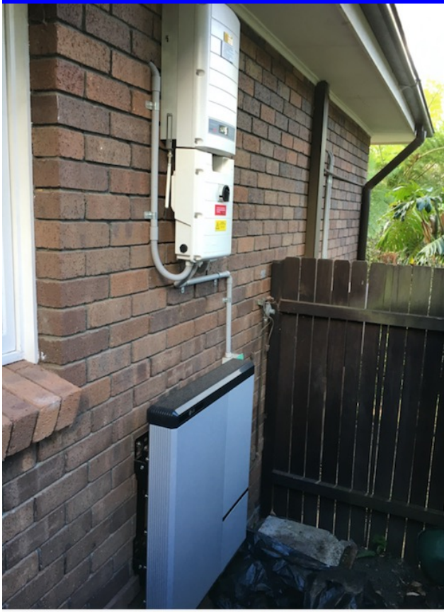
Domestic scale Battery below, inverter above
